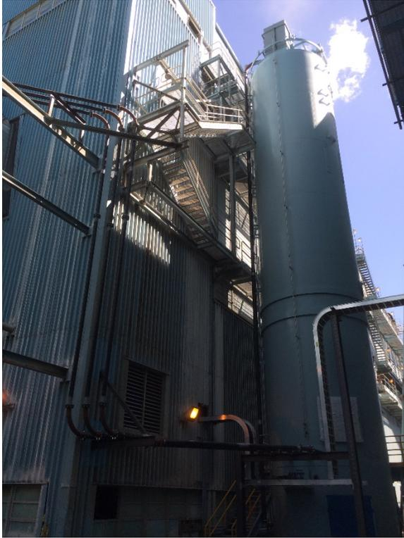
*Figure 9: ACI silo installed at LRS*
