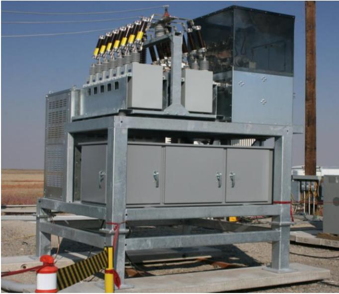
Figure 1 - Photo of the SolidGround™ Transformer Neutral Blocking System
