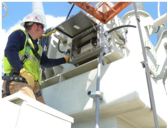
**Fig. 3** Sensor Cabinet Installation on an Autotransformer
