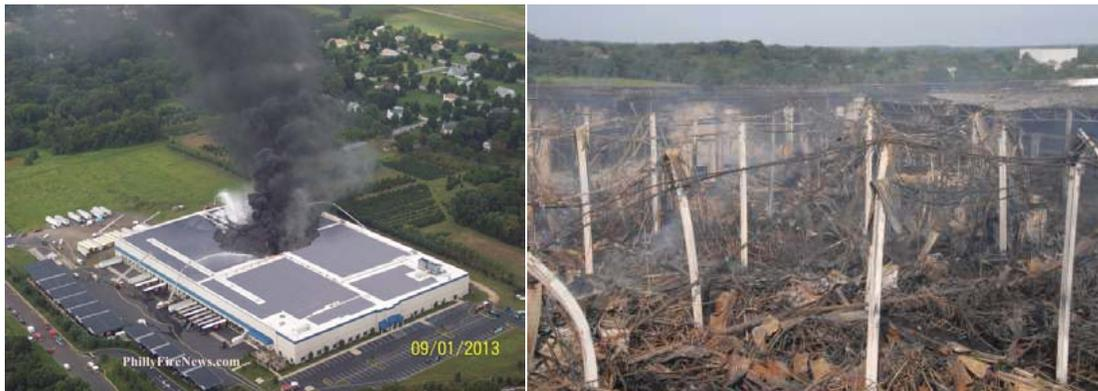
**Figure 6. Left image: an example of a building roof fire with a large conventional solar array. Due to the shock and flash hazards presented to the first responders (i.e., the inability to de-energize the PV system during daylight hours), the roof could not be trenched and the fire stopped. What would have been a roof isolated repair ended up resulting in a total loss (right image). Fortunately no one was injured in this event.**
