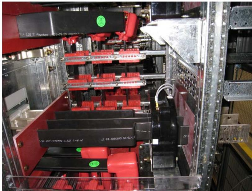
*Figure 11 – 480V Switchgear Insulated Bus and Zero-Sequence CT*
