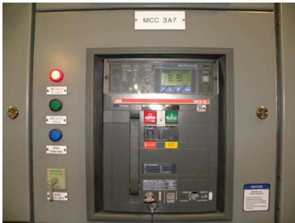
*Figure 9 – 480V Feeder Breaker*
