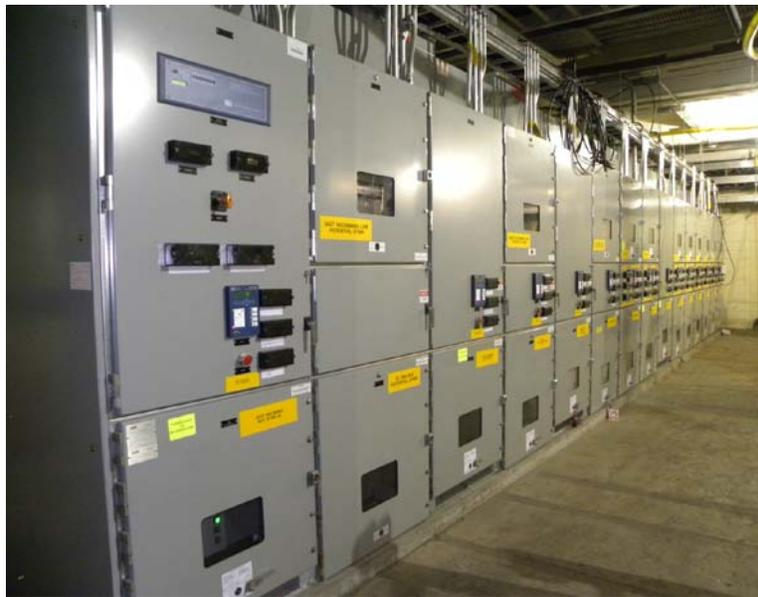
*Figure 4 –New Arc Resistant 4.16kV Bus 3A*
