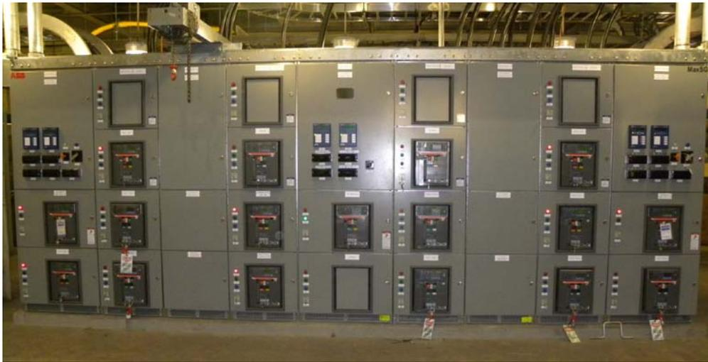
*Figure 8 –New 480V Metal-Enclosed Switchgear*
