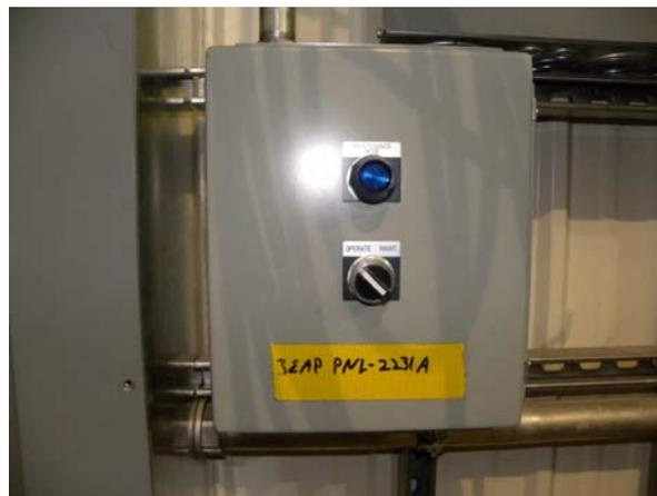
*Figure 10 – Maintenance Switch at 480V Panel*
