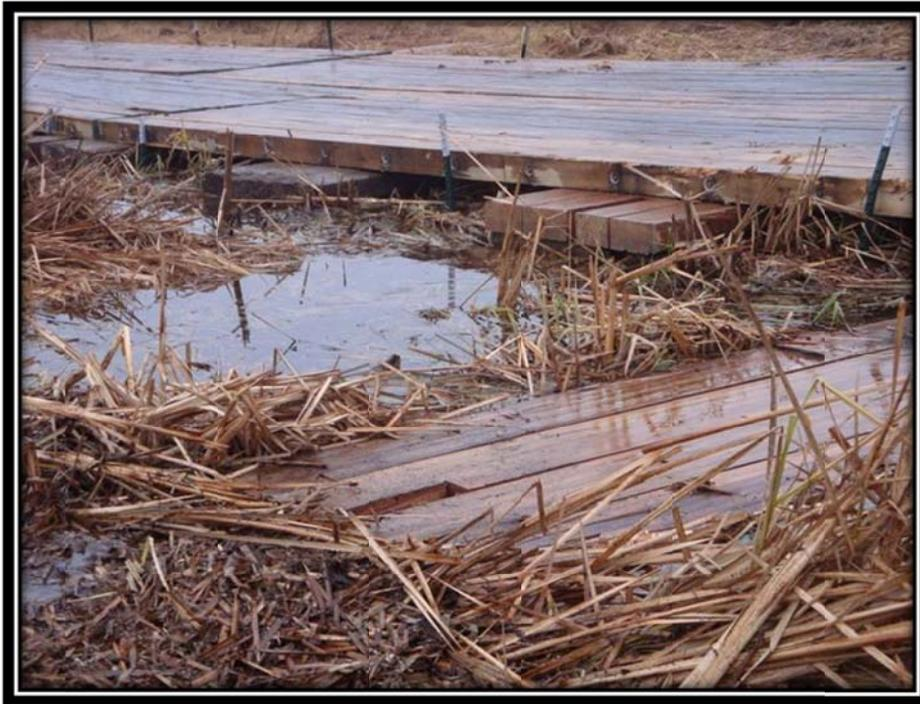
**Figure 3 -New South Mat air bridge system**
